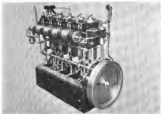
DOCK FIVE-CYLINDER SELF-STARTING MOTOR. †
